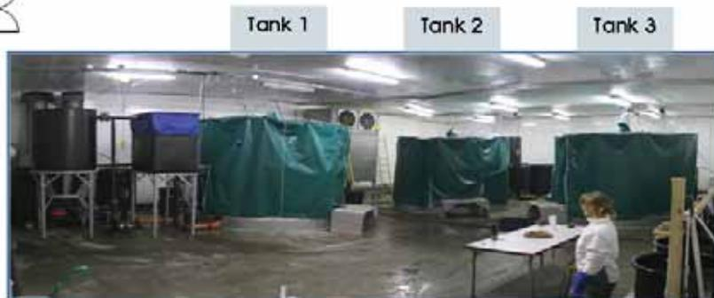
**Fig. 2.2.** Production hall, broodstock quarantine facility, Nexø. The production hall is isolated and cooled with a controllable cooling system. The three broodstock tanks (tank 1, 2 and 3) are thereby cooled as a result of room temperature. The lower half of the building is used for office, workshop, and storage for salt, tools and experimental tanks.
