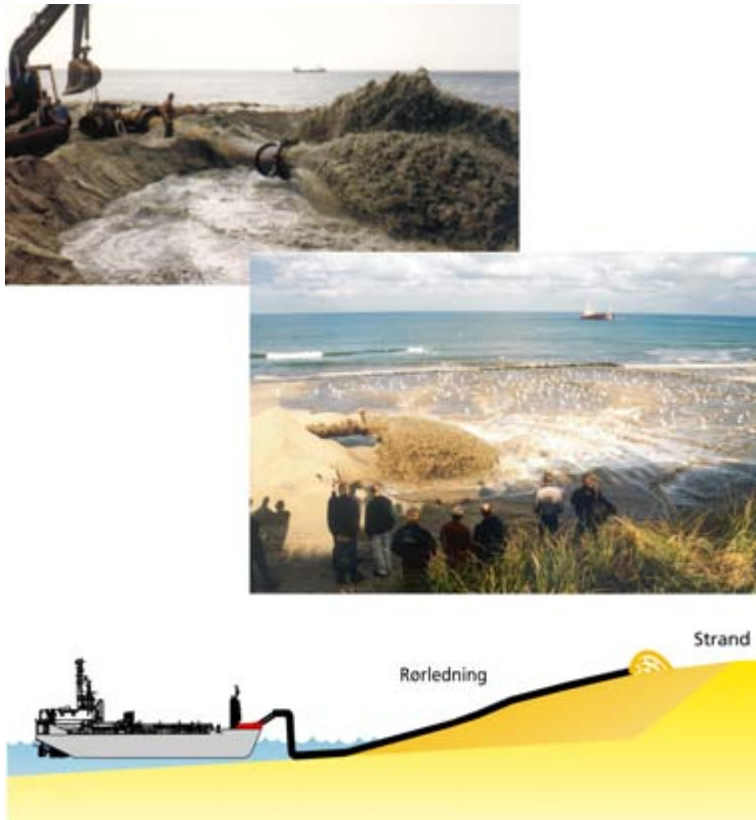
Figur 2.7. Princip strandfodring.
