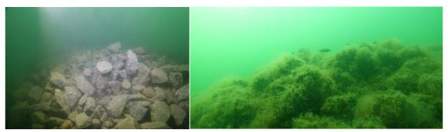
Figure 1.12. Pictures showing a newly deployed reef (December 2017) to the left, and the same reef surveyed in July 2019 to the right. About 1.5 years after reef construction, fish and macro algae increasingly occur on the reefs.
