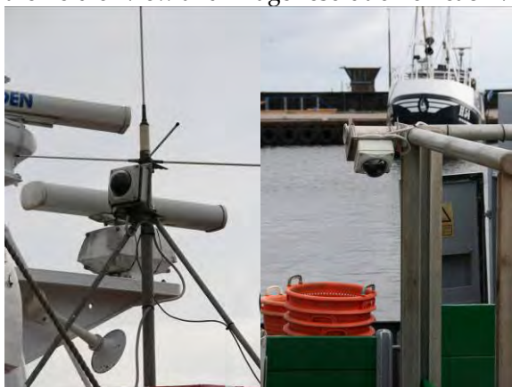
Figure 3. Photograph of an installed CCTV camera on a vessel encased in a cast aluminum armored dome.
