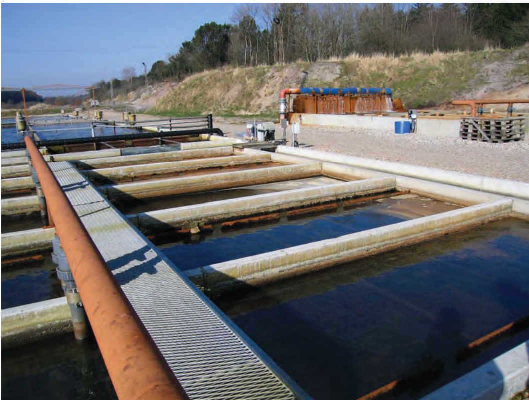
Figure 20. Biofilter divided into sections with bio blocks at Ejstrupholm Model trout farm (type 3). To the right of the biofilters is an ochre device for aeration of the abstracted ground water and precipitation of the ochre before the water enters the production units. Photo: Alfred Jokumsen.
