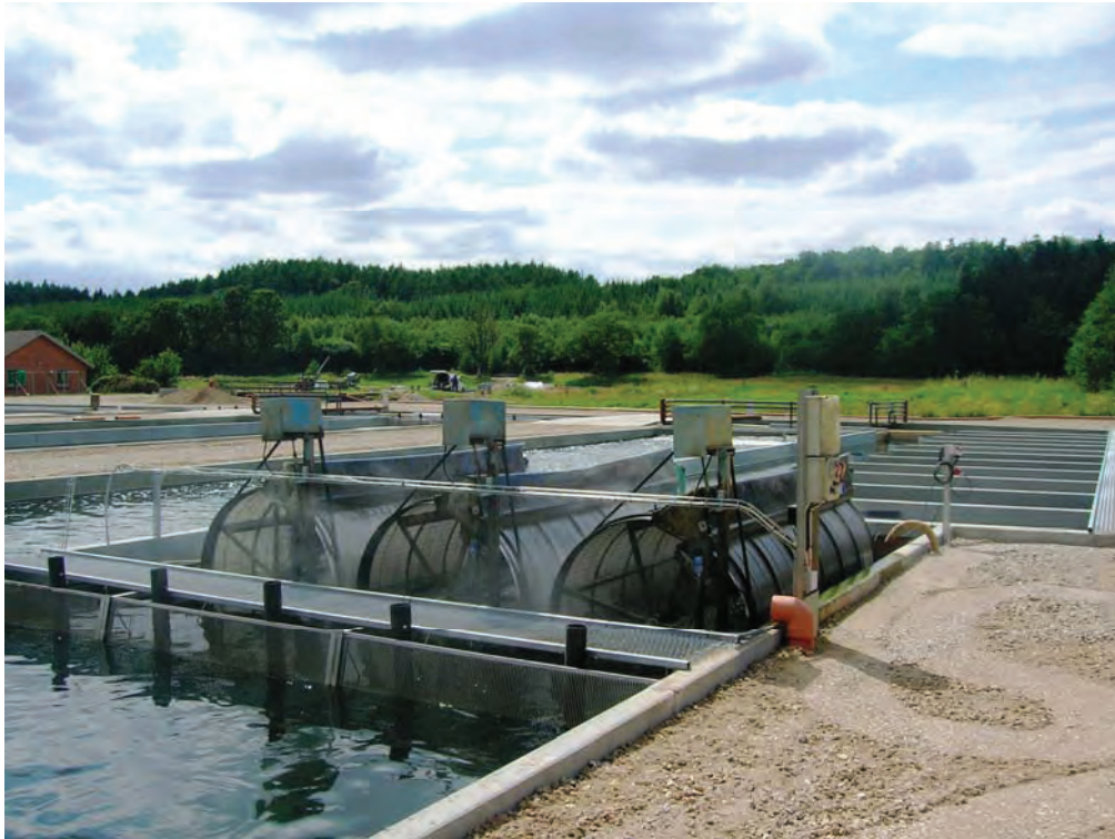
Figure 18. Micro sieves at Løjstrup Model Trout Farm (type 3). The micro sieves are placed just before the biofilters. Photo: Lisbeth J. Plesner.
