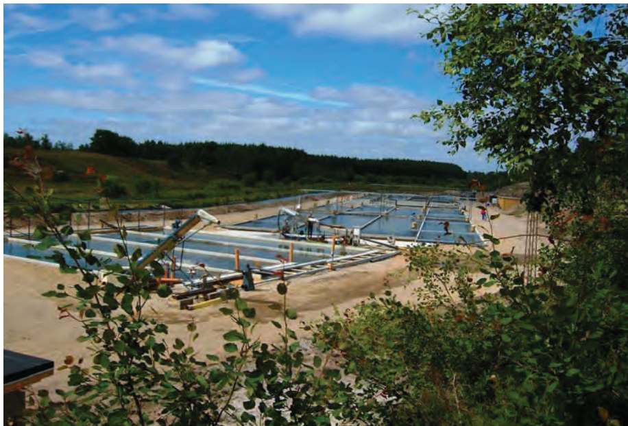
Figure 11. Ejstrupholm Model Fish Farm (type 3). The production units include two sections, each consisting of two concrete raceways. In the foreground, three concrete ponds for delivering fish are visible. In the background and to the left are the plant lagoons, which consist of the former earthen ponds overgrown with plants. Photo: Lars M. Svendsen.
