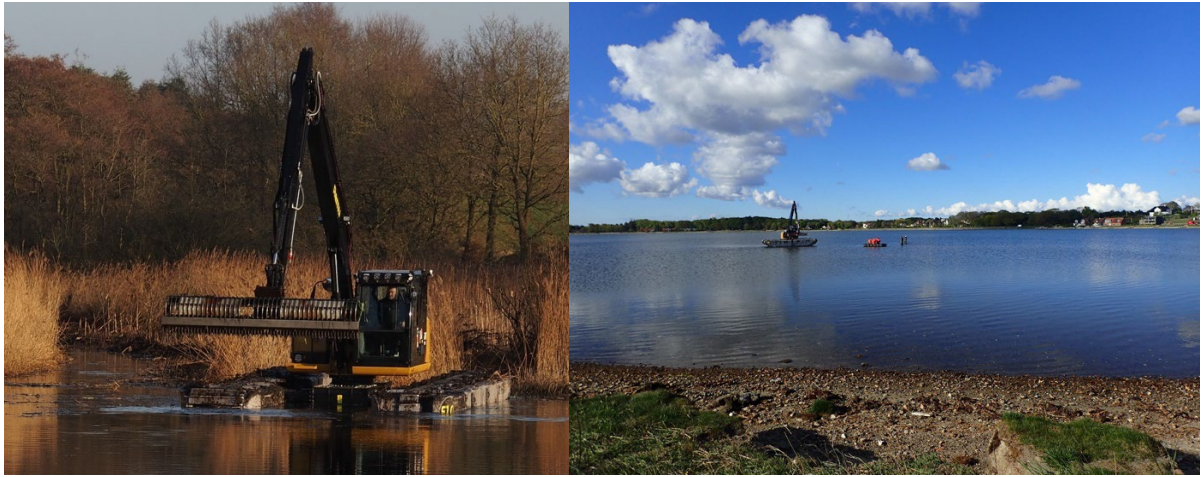
Figure 8.8.2. The E10 floating excavator (left) and sampling during the field trial in Klosterbugten in Mors, Limfjorden (right) (Photos: Sloths Naturpleje (left) and Pernille Nielsen, DTU Aqua).
